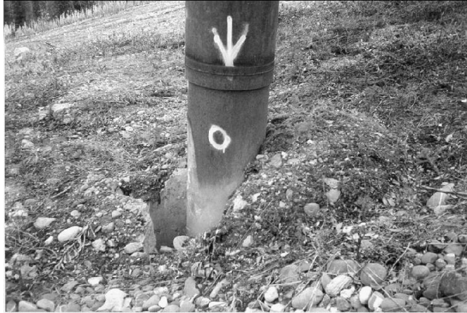
Figure 11. Mounding Around VSM
