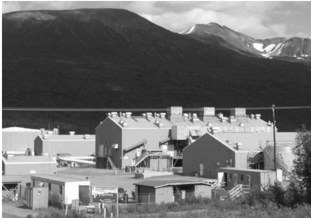
Pump Station 12, 65 miles north of Valdez, is the southernmost station.
